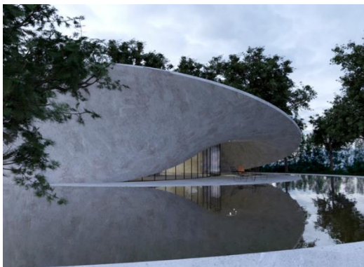
Slika 1 Mobius House of Hemp Bricks and Concrete (Antony Gibbon Design, 2024)
